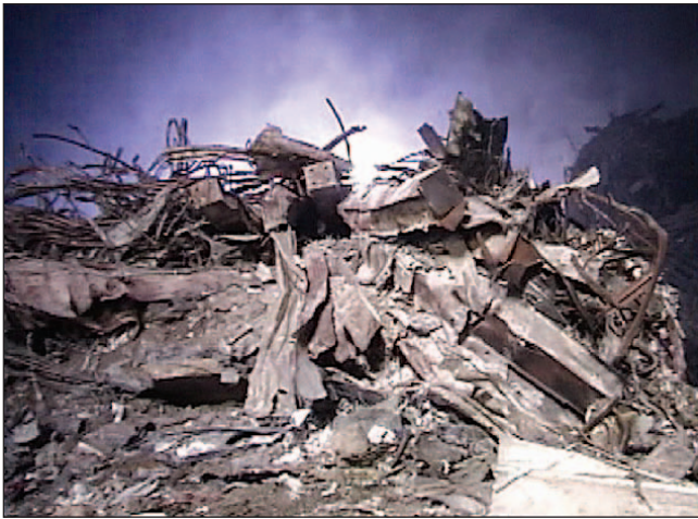
Figure 4. View of the rubble near WTC Tower 2 and Building 4 showing pancaking and the lack of voids.
